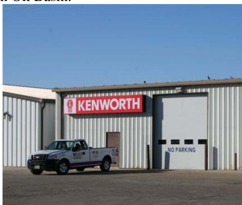
Wallwork Kenworth – Williston
